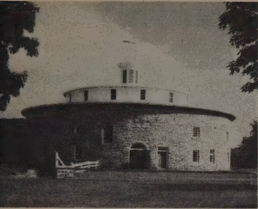
The Round Barn can hold about 400 tons of hay and 52 cows. Hay on top, cows in the middle, manure below. Gravity and biology combined.
